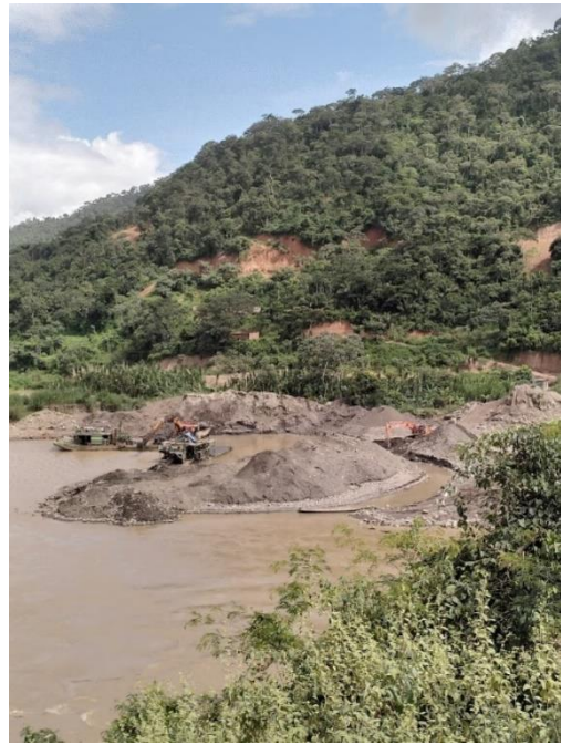
Figure 5: Visible obstruction of the natural river course at a mining site of cooperation Quillacas close to Teoponte
